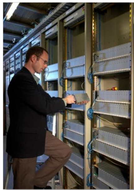
Our engineer inspecting the CRU Test Heads
